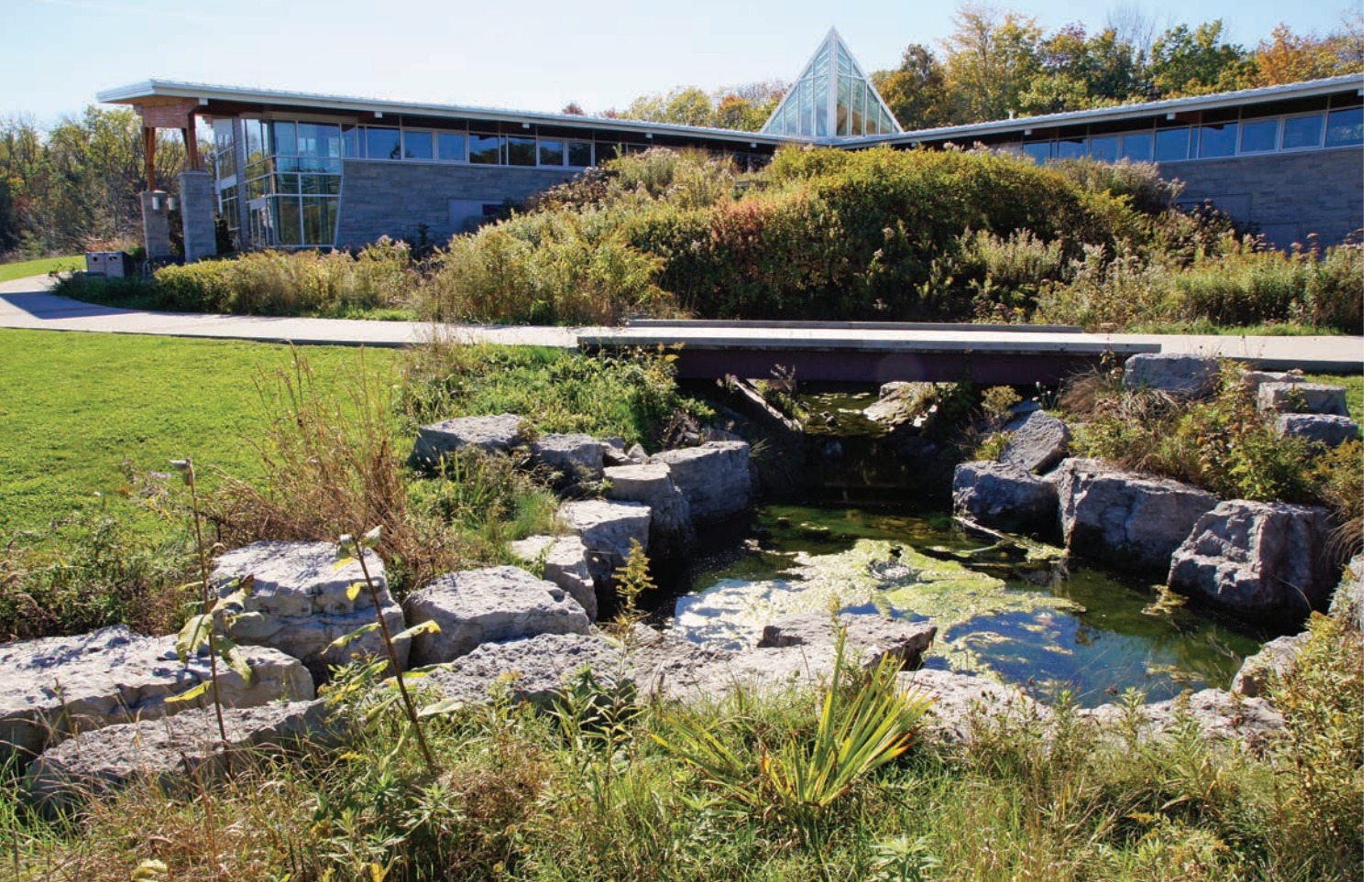
▲ The Centre for Conservation treats water carefully: cisterns store rainwater for dual-flush toilets, with excess rainwater feeding the natural pond surrounded by drought-resistant landscaping.
